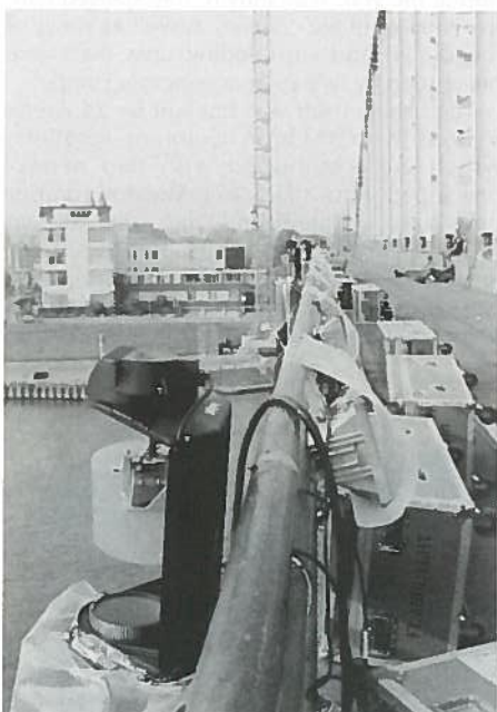
Super Scans on the bridge at Arnhem, with one of the 50m tall towers in the background.
