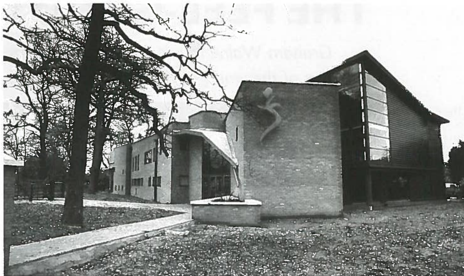
The Chicken Shed in Enfield: a steel framed auditoria contrasted with load-bearing brick supports.
