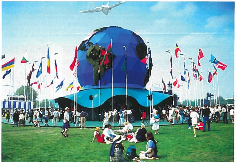
The Peace Globe, seated on a 12m revolve, supported by a ring of curved lighting truss and 12 truss columns, was constructed by Unusual Services, and rotated every 10 minutes.
