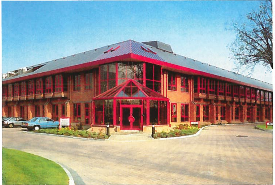
The impressive Hawley Mill headquarters of Electrosonic.
